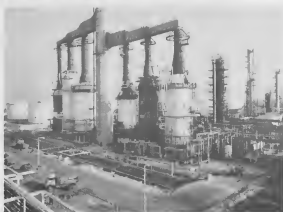
POWERFORMER UNIT, above, uses platinum catalyst in manufacturing high-quality gasoline. Tests necessary for control of production processes are performed in the refinery's modern laboratory, below. PLANTA AKI riba ta usa platinum catalyst den fabricacion di gasoline di alta calidad. Pruebanan necesario pa control di procesonan di produccion ta worde haci den e refinaria laboratorio moderno, abao.
